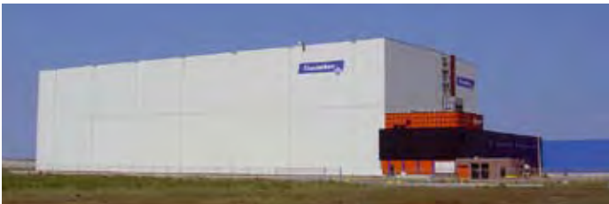
Freezer and cold stores
